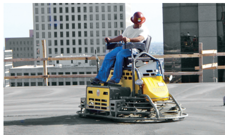
CRT 48-35L-PS Ride-on Trowel with Power Steer 48-in. ride-on trowel reduces the
