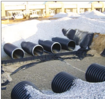
Due to impervious subgrade, cisterns and drain pipes were placed underneath to help collect the stormwater. Photo: Blake King
