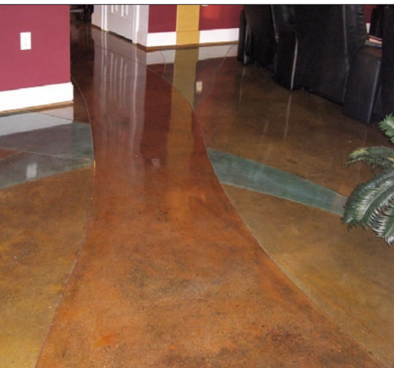
Floors throughout the house were acid stained and featured custom designs. Photo: Michael Osgood/AMT Enterprises LLC
