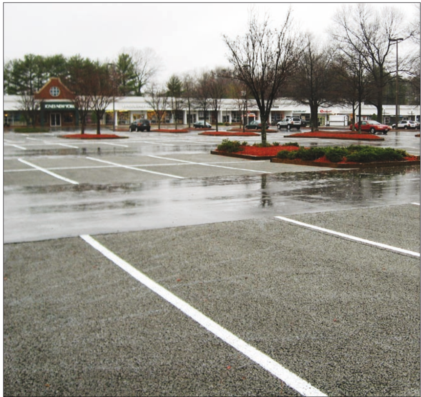
Williamsburg Prime Outlets choose pervious concrete for its parking lot replacement and expansion. Photo: Blake King
