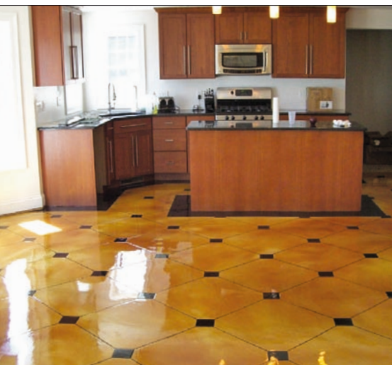
The small squares on the kitchen floor were hand-brushed with multiple layers of onyx-colored stain to reach a deep color. Black grout creates the tile look and coats of urethane create a shiny, glossy sheen. Photo: Michael Osgood/AMT Enterprises LLC
